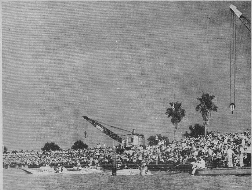
Two mobile cranes lifted the boats into the water over the heads of the crowd.
