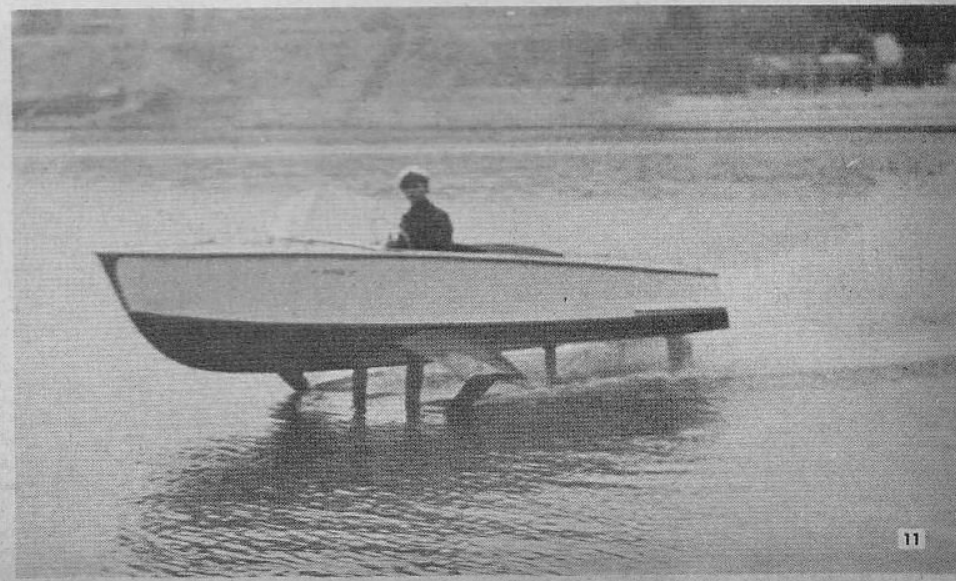
The first post-war German "Wing boat" at full speed. This is an action photo of a boat built from the open runabout design shown on the page of profiles. The gross weight of the finished boat was 1500 lbs.—power 30 h.p.—and the speed 37.54 mph. Note the minimum of water disturbance from this very efficient hydrofin.
