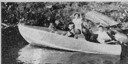
Feather Craft Deluxe Runabout, a round bottom aluminum boat. Length 13', Beam 59", Depth 29". Designed for motors up to 16 h.p.
