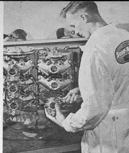
Mort Fife installing carburetors on the Square Six. Note gear box in position and dual manifolding which shows here.
