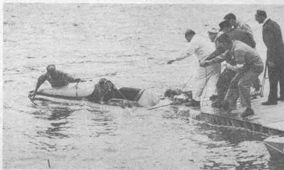
Gerband, a French competitor, aids in bringing in his disabled craft. Just after he won in Class X at the April Monte Carlo events, driver knocked a hole in the bottom of his boat. Gerband piloted a 6-cylinder supercharged Dupuy, which produced 100 hp, in overpowering his rivals.
