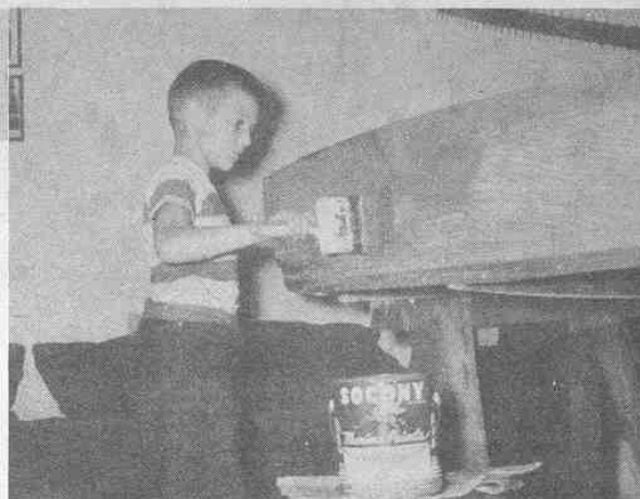
Craig elected to finish the hull with marine enamel over varnish. Sanding and painting were not included in 38½ hours of construction time.
