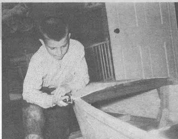
After a little practice, the builder learned how to use a block plane and was able to do all but the final finished fairing without help.
