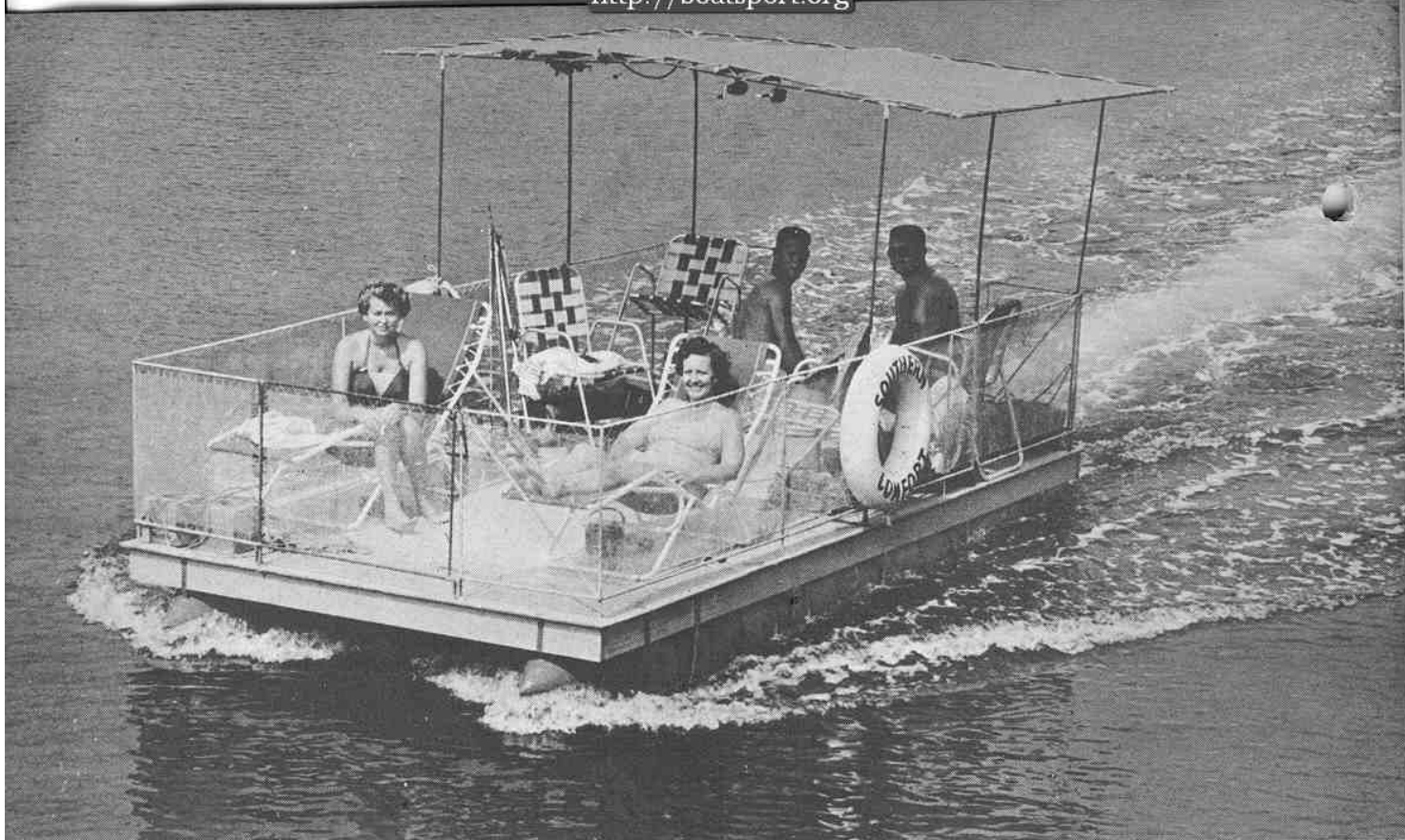
The Southern Comfort was built by Sonny Cooper and Pax Swartz, Sarasota, Fla., in their spare time for $100. Oil drums are used as pontoons.
