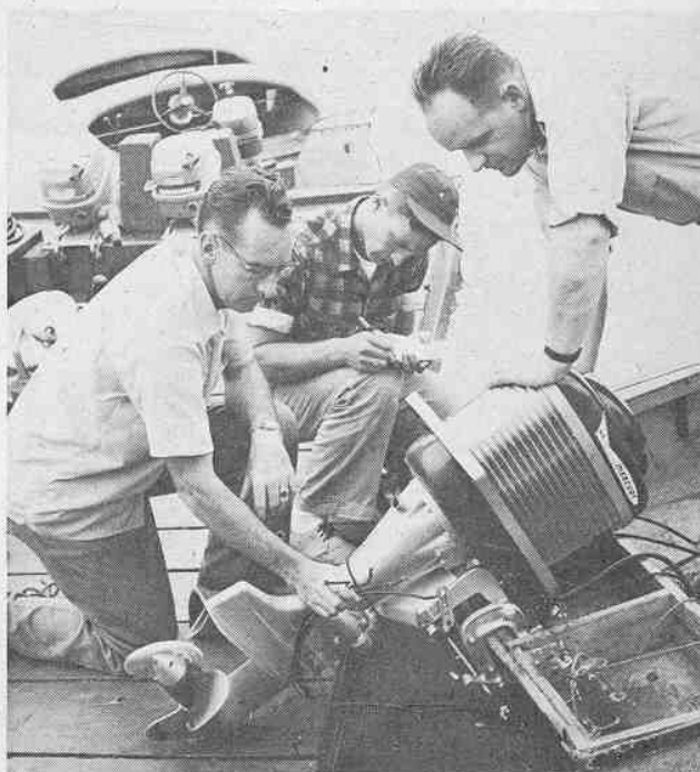
Jim Wynne, at left, shows how the shock snapped the steel-filled tie-down cables. New mounting bracket was intact after 102 passes.
