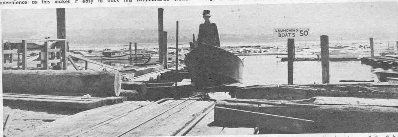
This launching ramp may look a bit rough and ready, but it's easy to use and you'll note that it is in a well protected place along the
