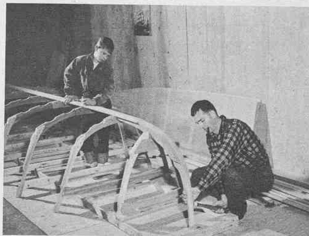
(Above) Frame is assembled upside down, with side of packing crate used as jig.
