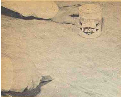
Be sure to fill all seams, holes and gouges with the non-oily seam filler. There's no need to fill hair-cracks.
