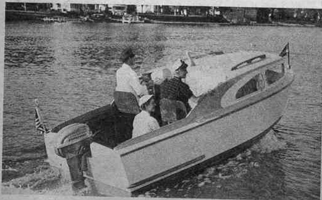
(Below) '54 Ozarka 18' kit cruiser has enlarged cabin, new lines and rounded windshield. Other kit models, 8 to 14', include stock racers and 12' Trailer-Boat that folds amidships to form own short trailer.
