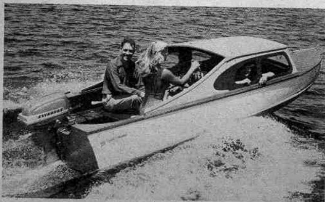
(Below) Day cruiser, like other Tomahawk boats, has either compression sealed or glass-covered hull. Small boats with cabins for shelter are becoming more popular for low-cost outboard camping-cruising purposes.
