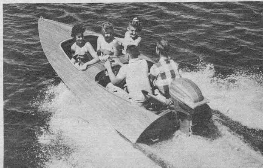
(Below) The Lightning 25, one of three family runabouts in Switzer-Craft fleet for 1953. Based on structural pattern of successful Switzer Bullet utility racers, this 12-footer has V-bow and 41" planing surface at transom; is designed for motors of 10 to 25 hp.
