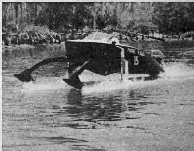
(Above) The Hydrofin becomes foil borne and even on choppy seas.
