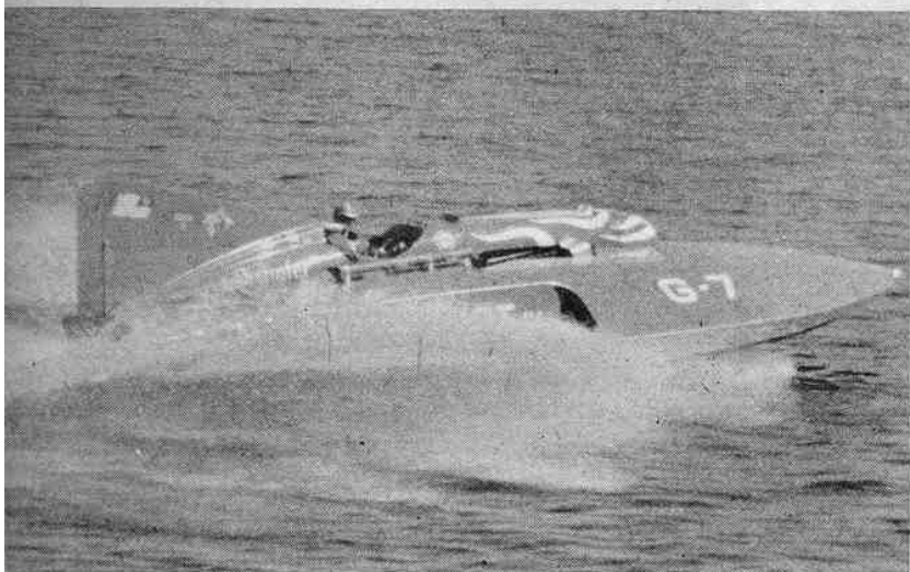
Bill Cantrell eases "Such Crust" around in preparation for 2nd heat. In this heat, on turn, boat exploded and burned. Prior mishap was thrown rod in qualification.
