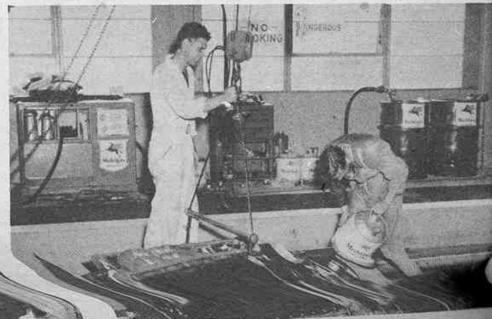
(Below) Stan Dollar (right) and riding mechanic, Howie Weeks, prepare "Skip-A-Long" for '49 Gold Cup. Cockpit of metal-skinned hull was amidships, unique among large speedboats but designed for greater strength forward, easier driving.
