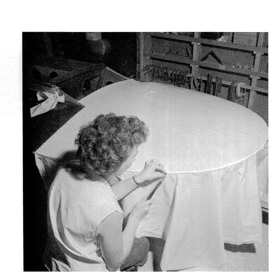
16. Fabric decking almost all tacked in position. Excess is later cut off. Remember to give this at least 6 good coats of dope, prior to painting.
