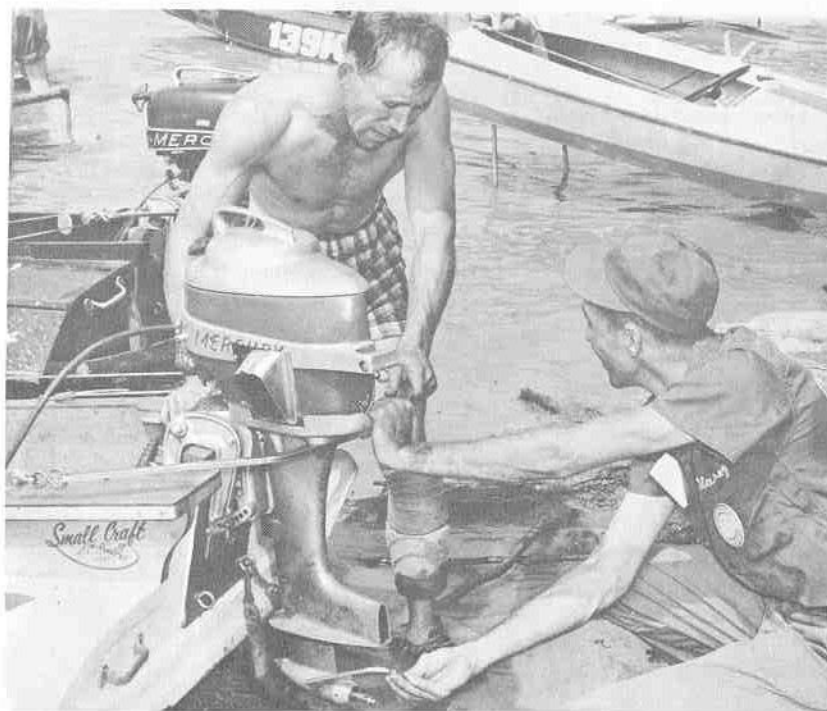
N.O.A. Inspector Bud Harvey checks the lower unit measurements of the Mercury 20H helmed by Ralph Scott, Paducah, Ky. Though Scott finished third with this rig, his modified Mercury A. carried him to an N.O.A. Division IV hydro title.
