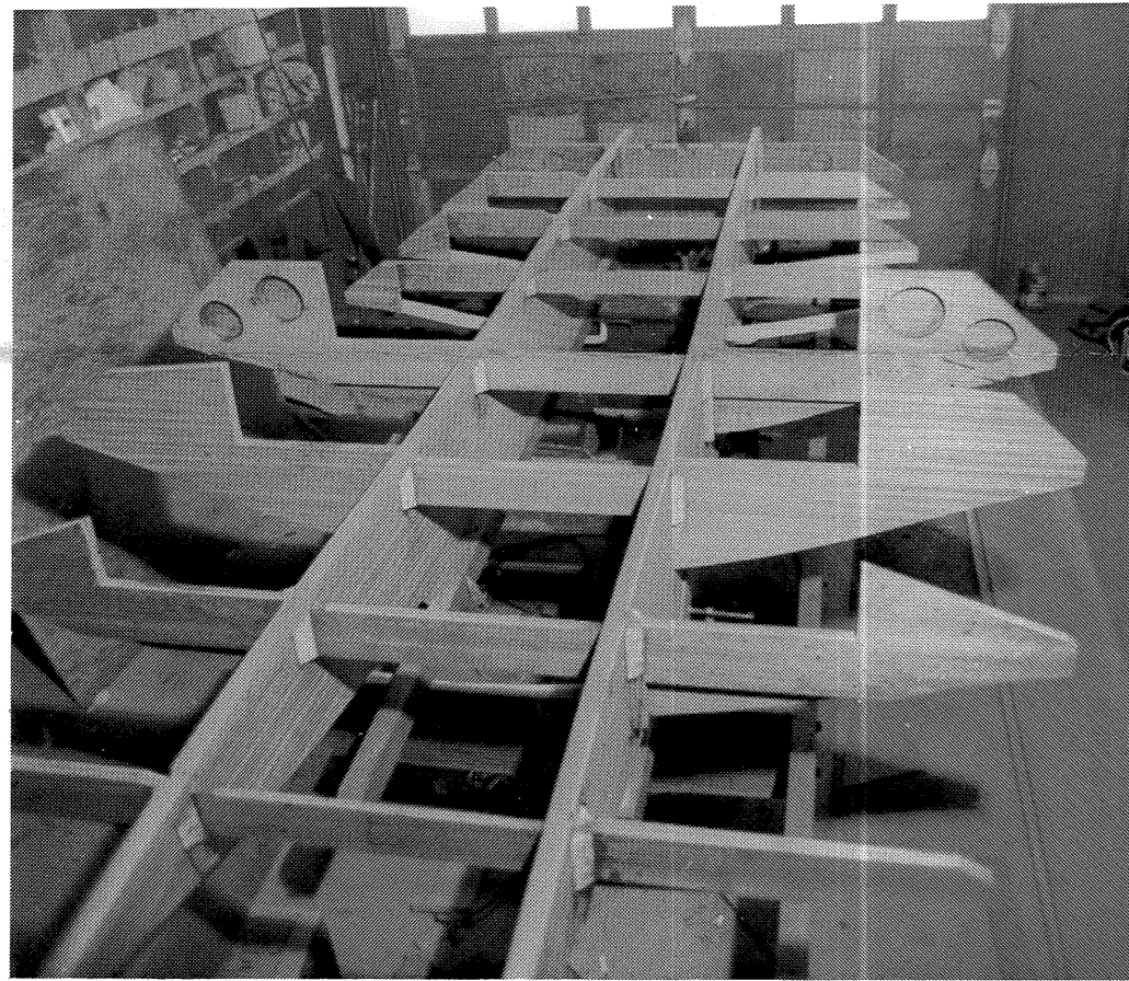
7. All ribs are in place, except the transom. Note that two battens are glued and nailed to the girders and screwed to all ribs.
