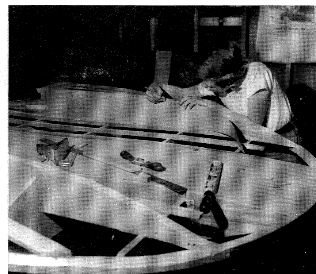
23. The after plane is added to the sponsons which are carefully trimmed to size. Take the measurements off the rib drawings. After one is done, trace on to a piece of stiff paper and mark off this shape on the other sponson so that both sponsons are identical.
