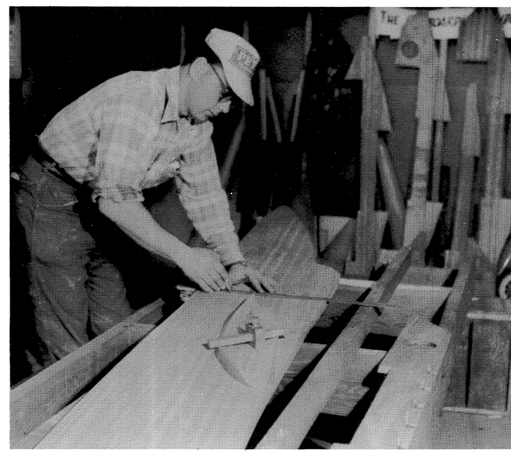
4. Both girders are temporarily fastened together. Slots for ribs are carefully marked off and cut out.
